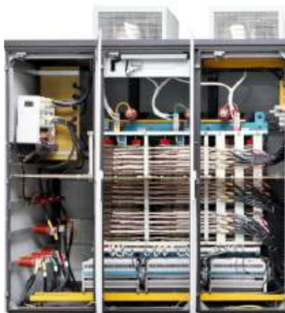
Fig 3.6 Layout in the transformer cabinet
