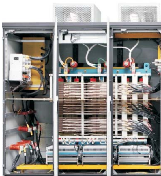
Fig 3.6 Layout in the transformer cabinet
